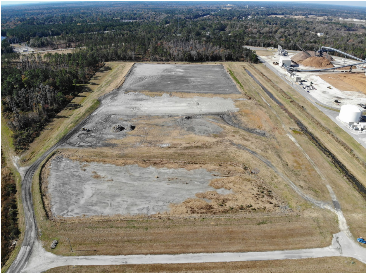
Figure 2. Aerial Image of CCR Landfill Facing West
