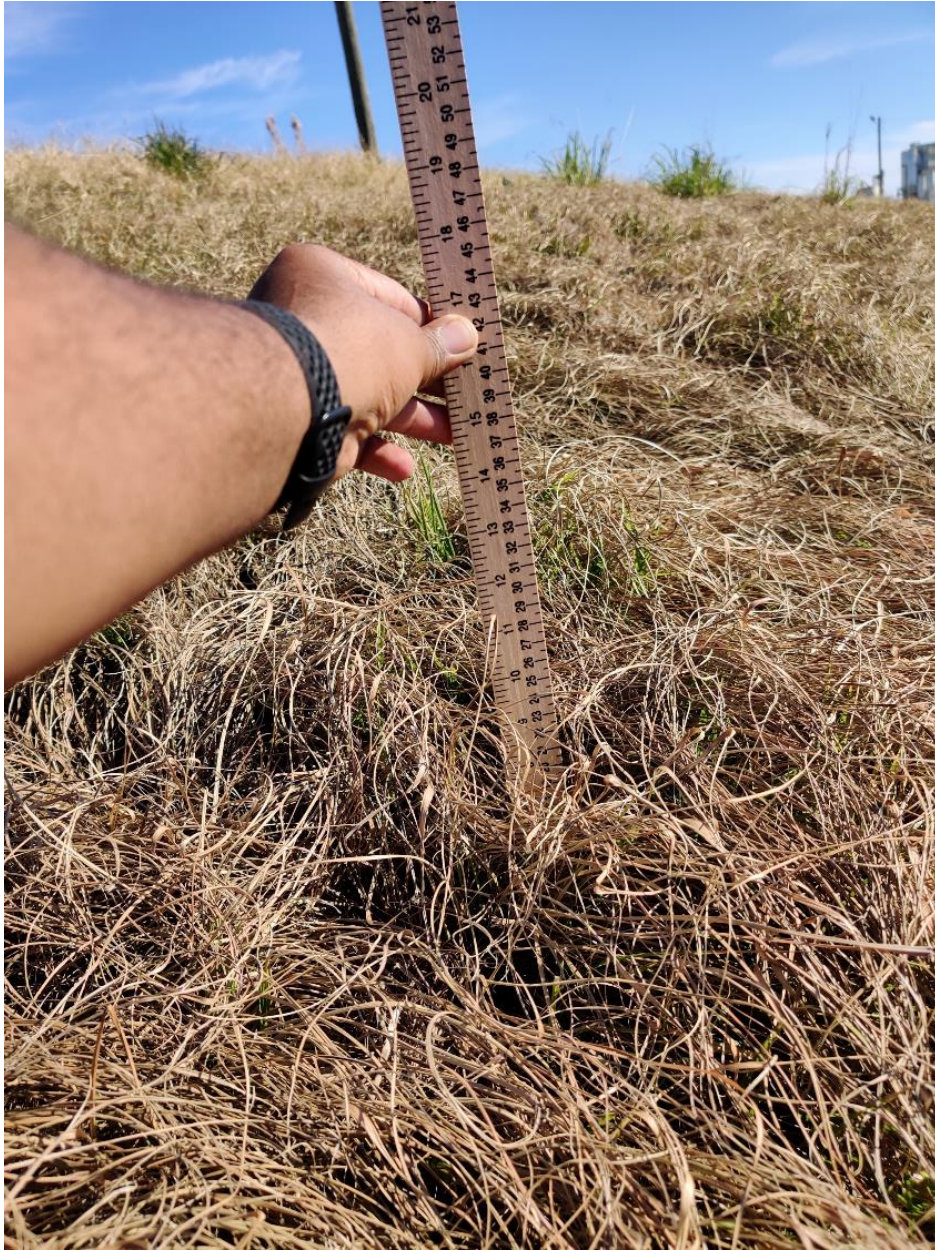
Figure 6. Grass Height Greater than 6 inches Observed on External Slopes of the Surface Impoundment System
