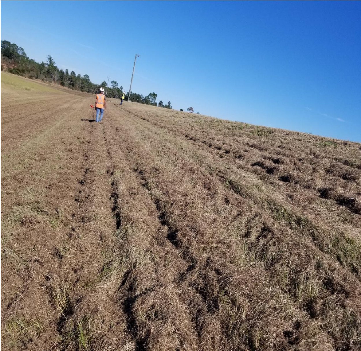
Figure 7. Accumulated Grass Clippings Observed on the External Side Slopes of the Surface Impoundment System
