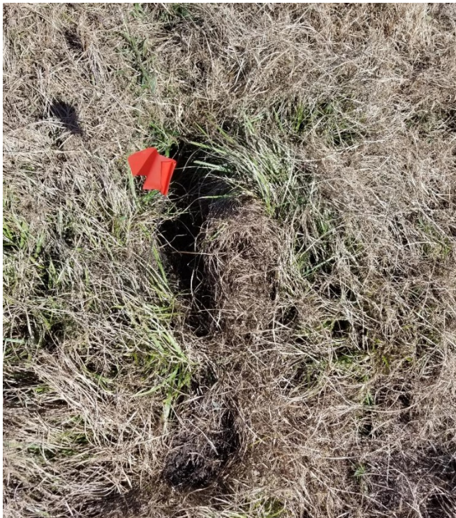
Figure 5. Forage Hole Observed on External Slope of the Surface Impoundment System
