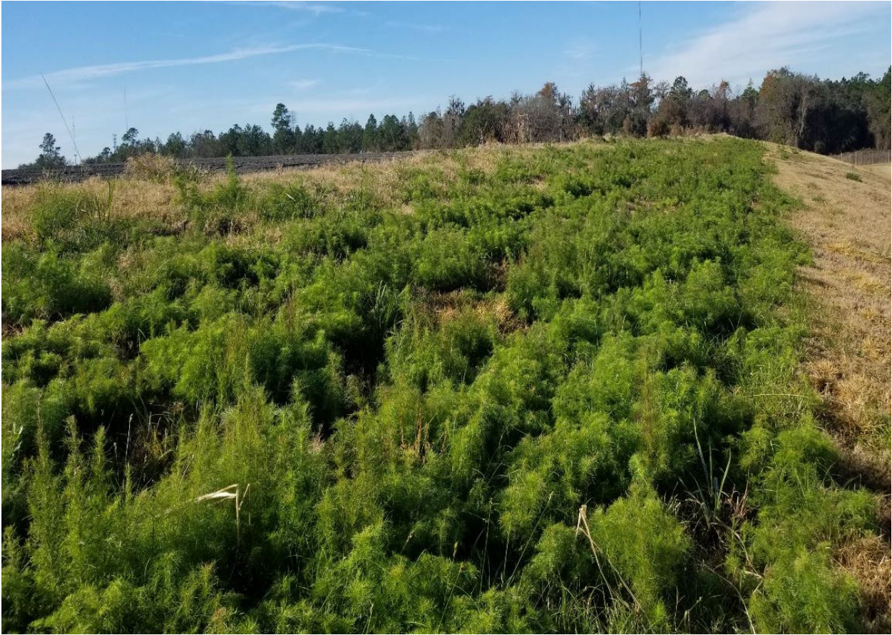
Figure 9 Patches of Tall Weeds on the Northern Slope of CCR Landfill
